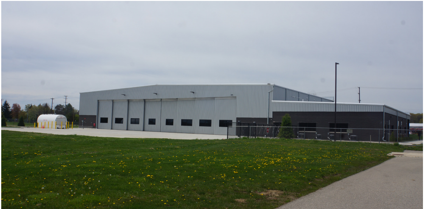
One of the highlights of the project is the 110' x 20' sectional power sliding hangar door with 8' x 4' windows in each panel.
