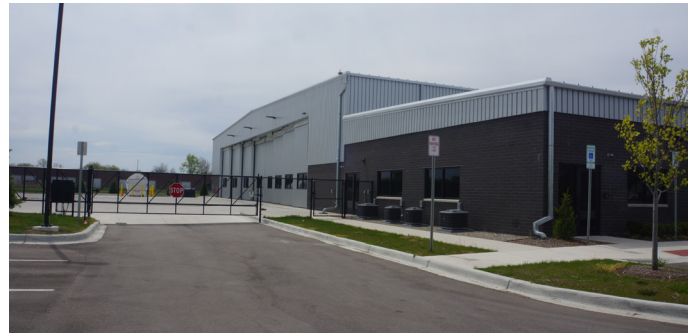
The exterior walls of the building are 8'-high masonry using 4"-high color block.
